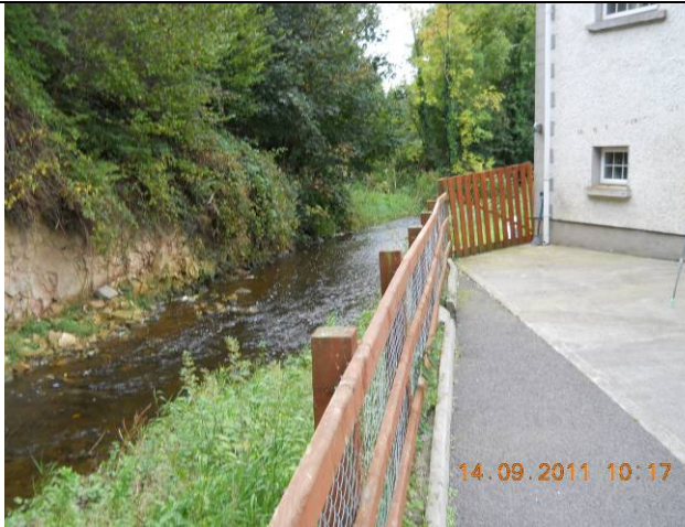
Property downstream of Bridge has history of flooding
